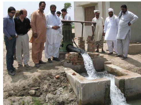
USAID is funding the installation of more than 11,000 new tubewell pumps
