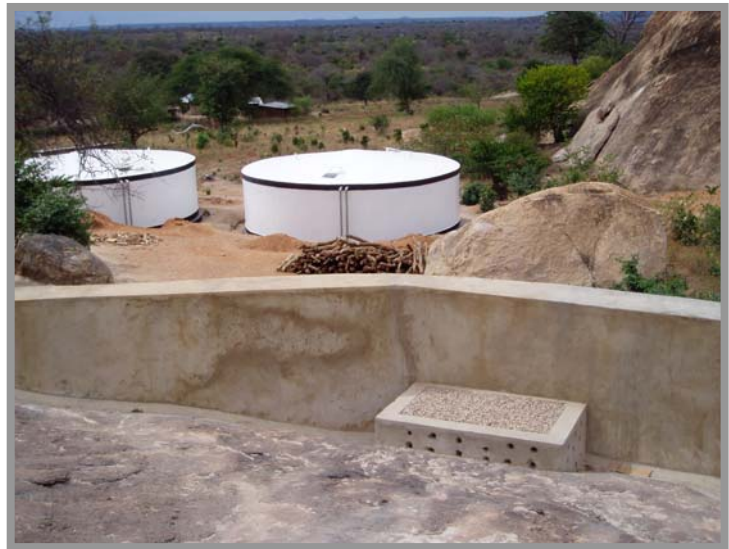
The basin of Muliluni Rock Catchment in Makueni District, Eastern Province, collects rainwater to fill the storage tanks below (Courtesy of WHH).
