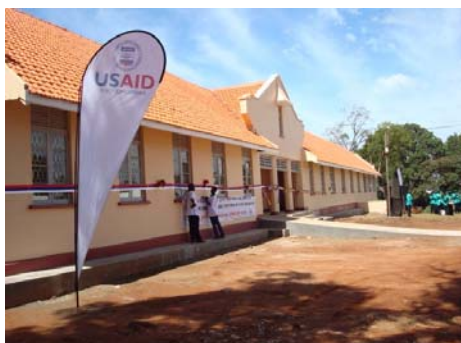
The reconstructed offices of the Resident District Commissioner in Gulu.
