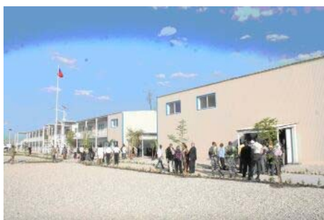
Officials gather for the inauguration of Haiti's temporary Parliament buildings.
