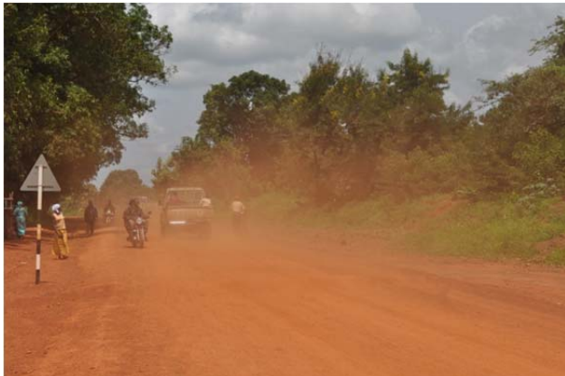
Vehicles, motorbikes, and pedestrians share this road in Western Equatoria that USAID improved to all-weather standard. Photo: Sarah Armstrong/USAID
